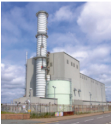
Great Yarmouth Power Station
